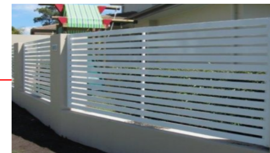
HORIZONTAL POWDER COATED INFILL SLATS FENCE
