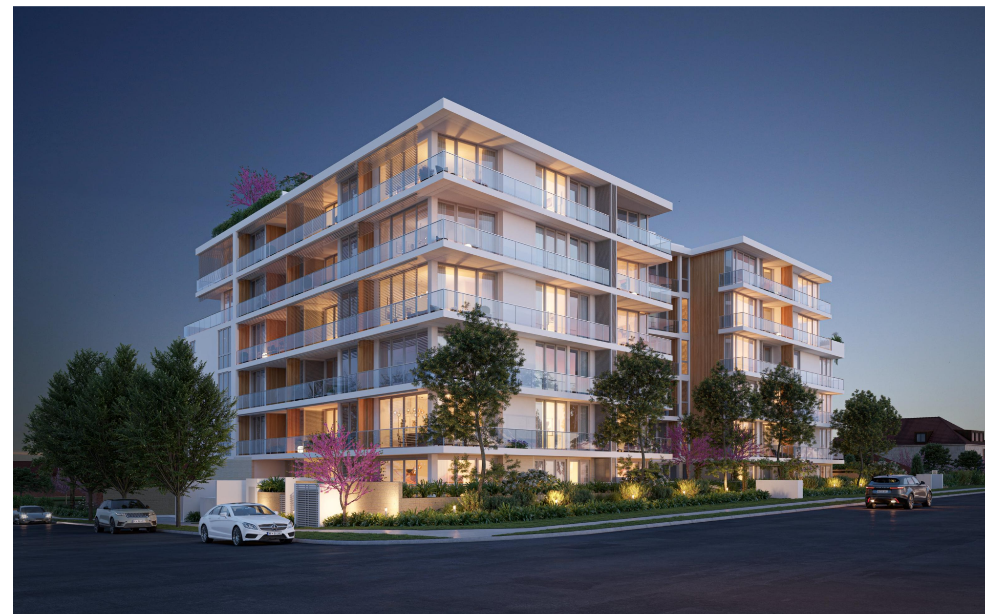
VIEW FROM CORNER OF NEWTON ROAD AND CARINYA STREET
